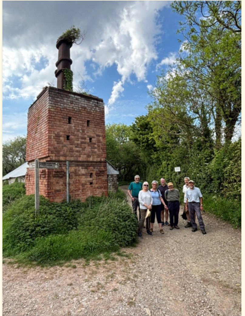
Members of the Geology Group at the disused retort (a device for distilling crude oil) at Kilve, north Somerset.
